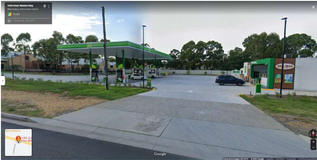
Figure 7: The station after upgrade
